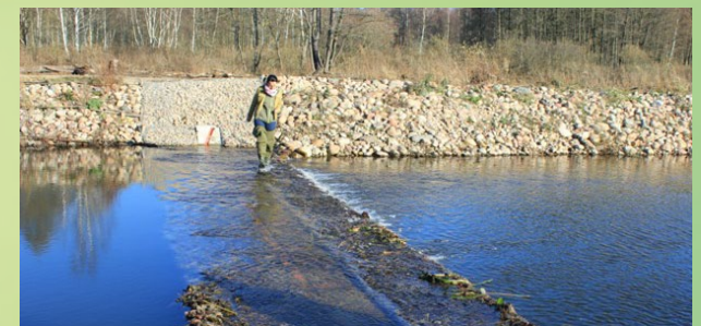
Water threshold built on the Woźnawiejski Canal
